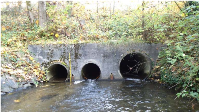
City of Burnaby culvert, photo courtesy of Opus DaytonKnight
